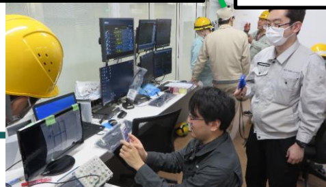
First Beam in Treatment Room
