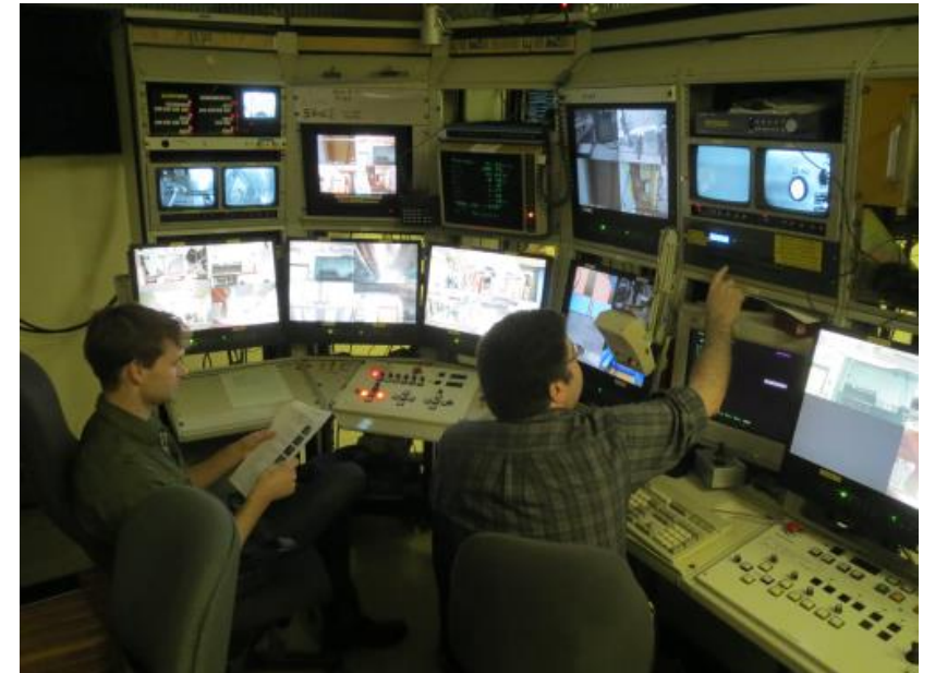
RH cyclotron control room
